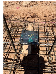
Column Footing Rebar
