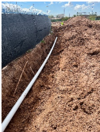
Relocated 4" Irrigation Line
