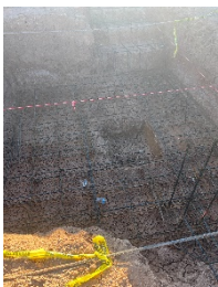
Elevator Pit Rebar
